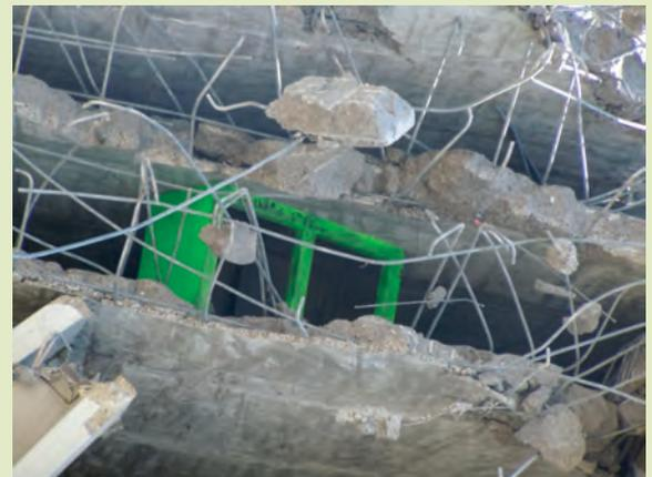
*School desk placed on the 6th floor during implosion. Four concrete floors pancaked down on top, but they were no match for the strength of the desk. The desk held the 6th and 7th floors apart with no deformation.*
