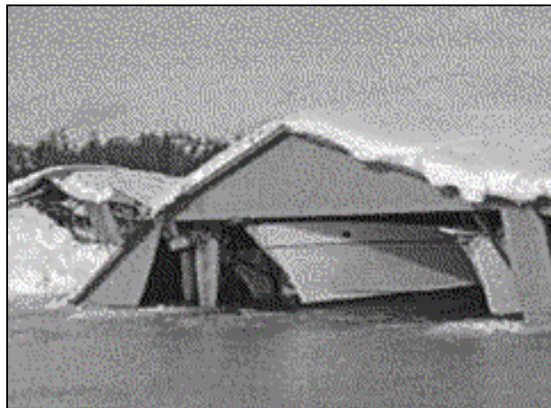
Boat houses in Sidney and North Saanich collapsed under the weight of snow
